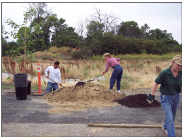
Mixing the backfill at Coyote Creek.
